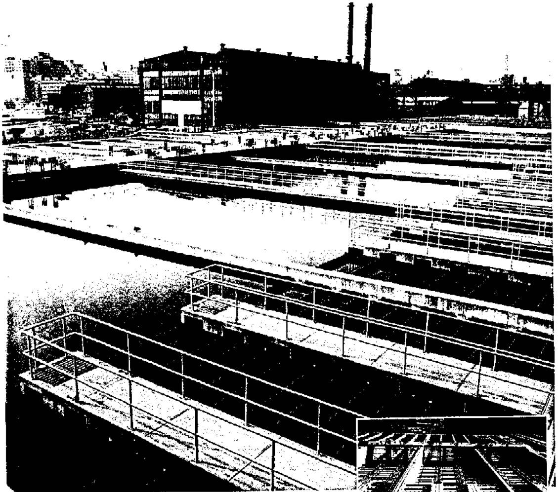
Above: Final settling tanks, where the solids are settled and removed. Right: Empty final settling tanks, showing collector mechanisms, which are used for collection and removal of settled solids.
