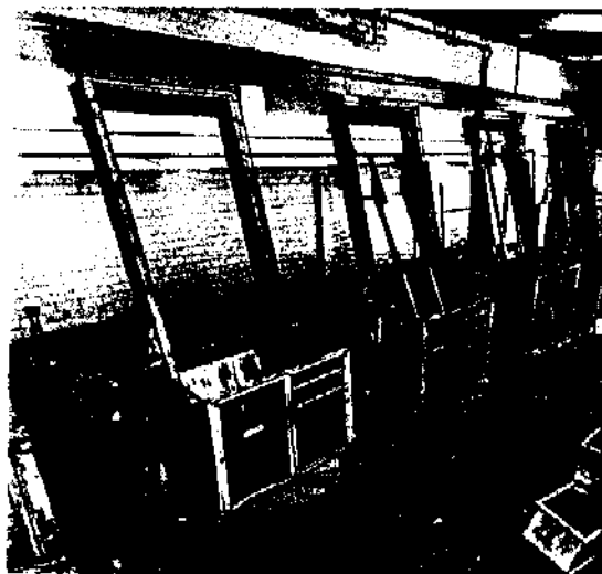
Bar screens remove the large solids and debris from the wastewater.
