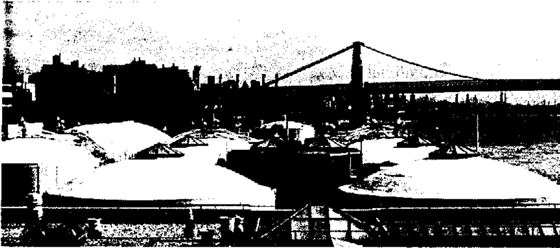
Above: Overall view of the solids handling facilities, including the thickeners, digesters and sludge storage tanks, with the Williamsburg Bridge in the background.
