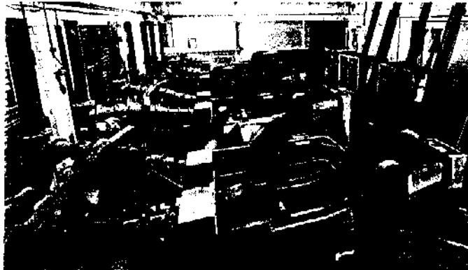
Right: Degritters remove sand particles from the settled solids, or sludge. This type of separator was originally patented for placer mining, the separation of gold from the settled particles of sand.
