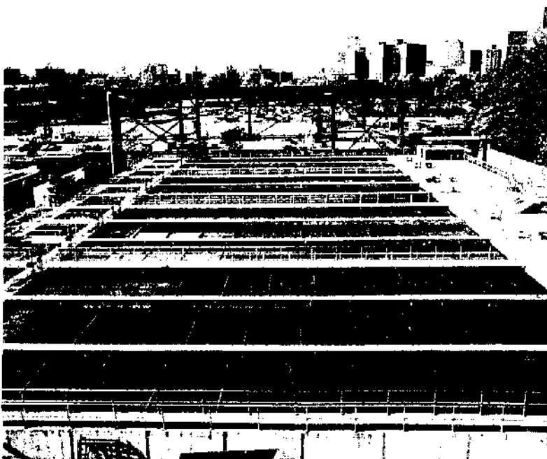
Final plant effluent overflowing the chlorine contact tank weirs.
